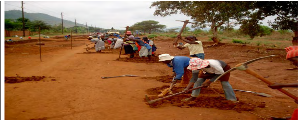
Picture 5: Labour intensive methods create jobs and ensure skills transfer to communities
