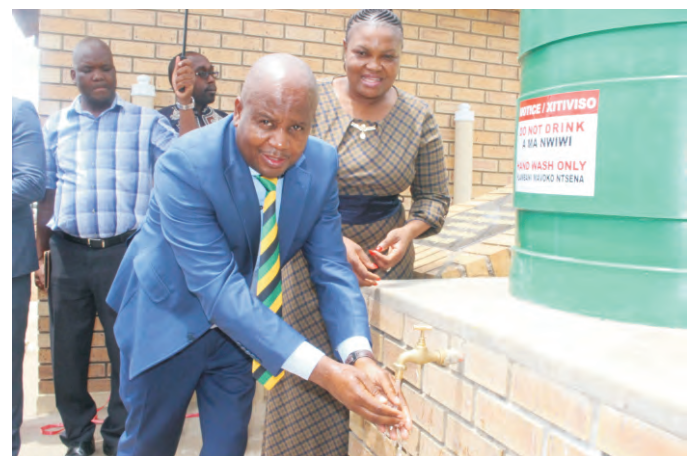
MEC Makamu washing his hands outside the fully-fledged ablation facilities at N'wamankena.
